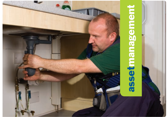
UPP's maintenance staff at work at Loughborough University
