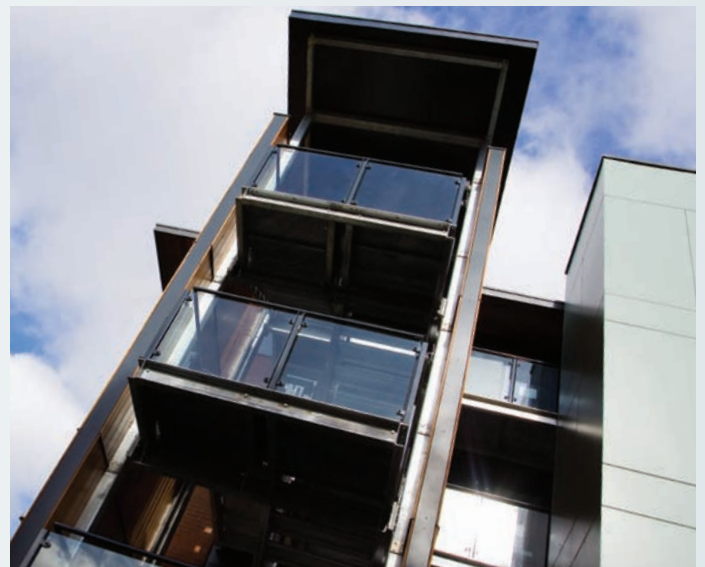
Fire escape stairwell at UPP's Carnegie Village
