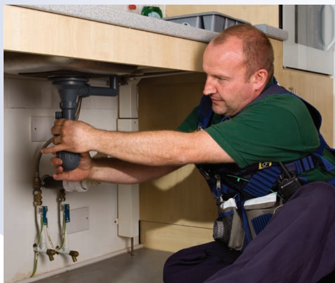
UPP's facilities management services at Loughborough University
