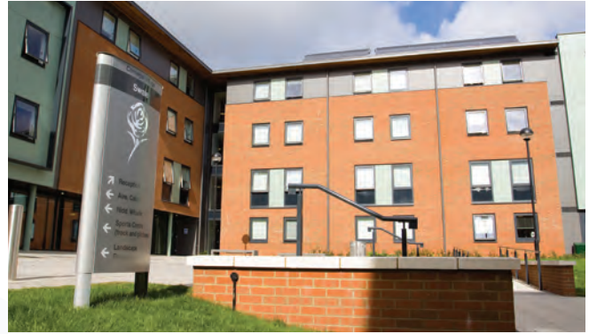
UPP's award winning £26 million scheme at Carnegie Village, Leeds Metropolitan University was built to PassivHaus standard and provides 479 rooms
